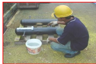
First coating with Rust Contact V Finishing with Aqua Sealer
