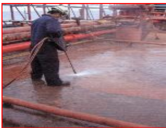
High pressure washing of the deck
