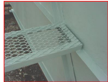
Rusted Surface after application of Rust Contact V
