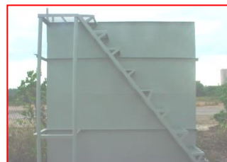
First coating with Rust Contact V Finishing with Aqua Sealer
