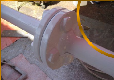
Application with Polyurethane (PU) for UV Protection
