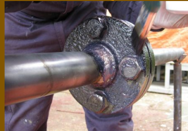
Contact V application as primer coat
