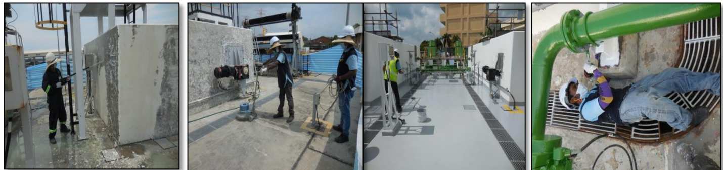
Stripe coat application-PU
