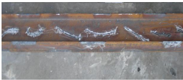
Before application of Aqua Filler
