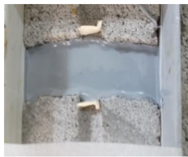
After application of Aqua Filler
