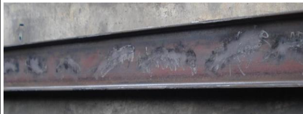
After application of Aqua Filler
