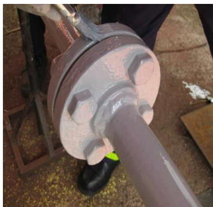
Aqua Sealer second application (External surface)
