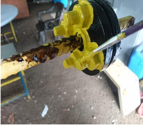
Aqua Edge application on the edges of Flange, Bolts & Nuts
