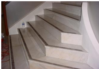
Anti skid system attached on the existing stairs in five star hotel
