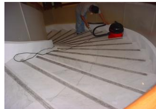
Anti skid system attached on the existing stairs in five star hotel
